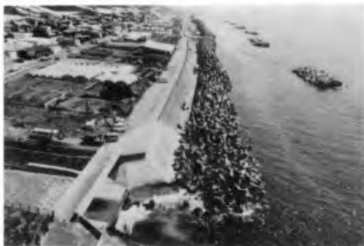
**Photo.2** Coastline totally covered by seawall and concrete armor units on the Shimizu coast. This picture was taken in July, 1995. The river flowing into the sea is the Takigahara River, which separates the Shizuoka and Shimizu coasts. These coastal structures were built to protect farmland just behind the seawall.
