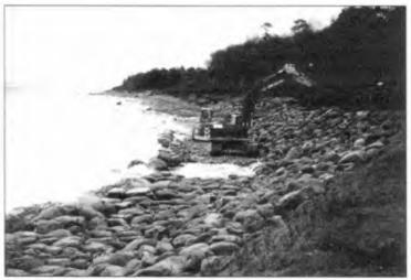
Figure 6 - Placing of geotextile and armour.
