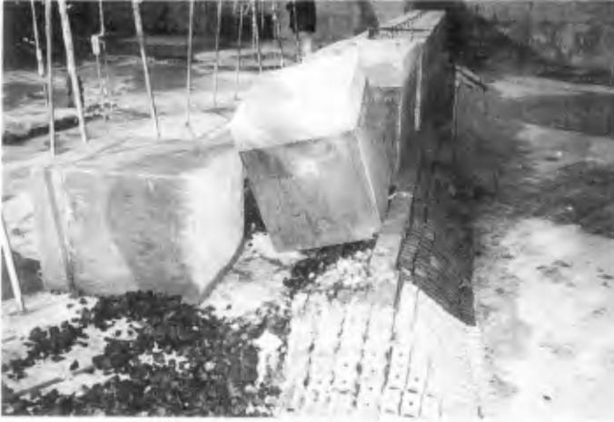
Photo 1. Damaged Caisson and Mound of the Outer East Breakwater
