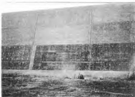
Photo 1(b) Air blow occurring from a gap between the caisson and backfill stones.
