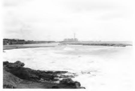
Fig.7. The first from the south of detached breakwaters and the tombolo
