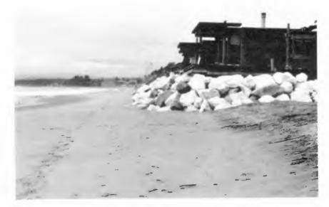
Figure 7. Early winter conditions. Berm has retreated behind revetment leaving uniform planar beach in front of revetment and control beach.
