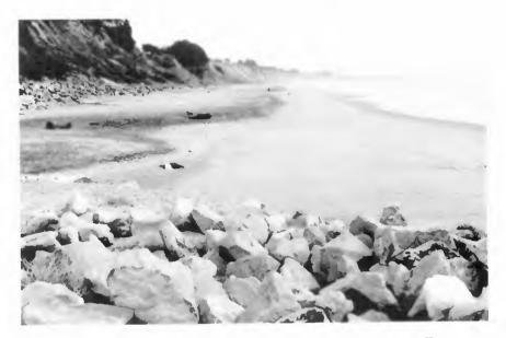
Figure 9. Localized scour adjacent to downcoast end of seawall.
