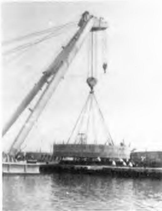
Fig. 5. Cylindrical caisson fabricated on quay apron.
