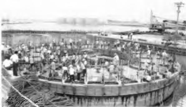
Fig. 4. Cylindrical caisson fabricated inside the dock.
