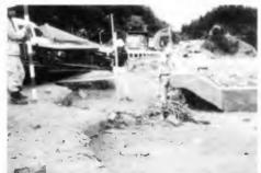
Photo. -2 Destroyed seawall and road due to storm surges (Sosu coast, Typhoon T8613)
