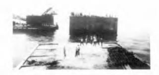
Figure 8. Installation of an "Island" caisson, which is aided by a pre-anchored 80 MT pontoon
