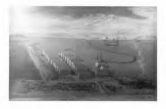
Figure 3. Caissons made on the beach where is dredged for harbor basin later
