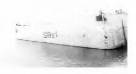
Figure 6. Caisson slides toward water under process of Slide-to-Float method
