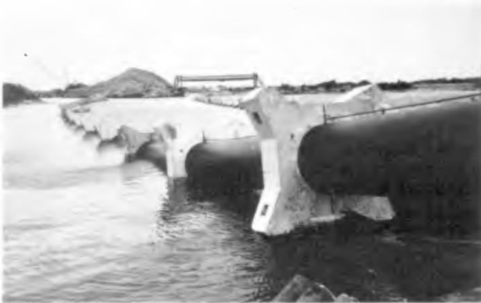
Figure 1: Typical star weights, Richards Bay HDPE pipeline
