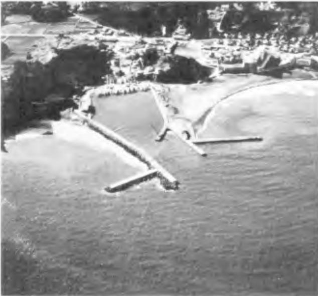
Fig. 5 Recovered Taito Harbor after rip current barrier construction.
