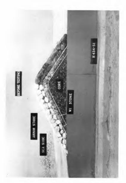
Figure 2. Cross-sectional view of typical stone section.
