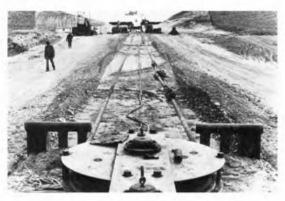
Photo 1. Pipeline Pulling of the Flags Gasline at St. Fergus.
