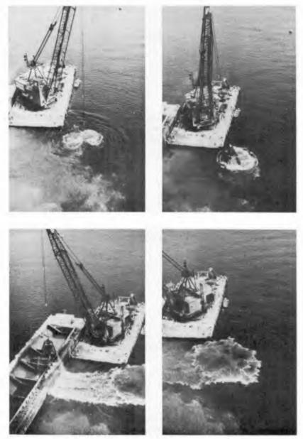
Fig. 7. A typical dredging sequence - beginning ascent upper left - residual wake - lower right. Thames River 1977 - 1978.
