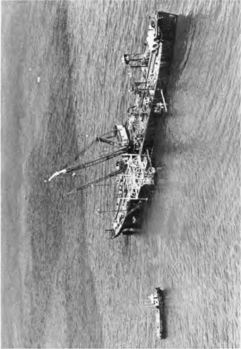
Fig. 9. Pipelaying Barge Used in Construction of Sand Island Outfall.
