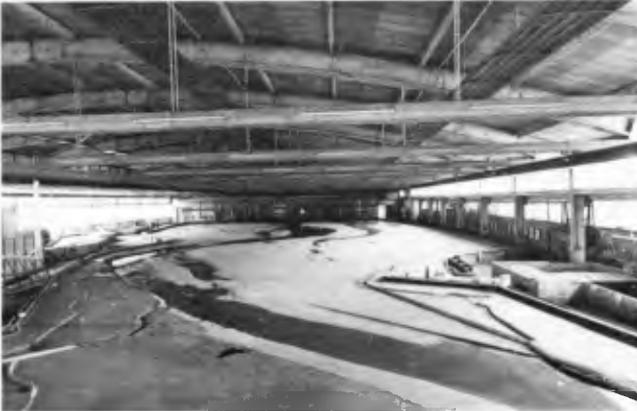
Fig. 2: The Elbe model with moveable bed
