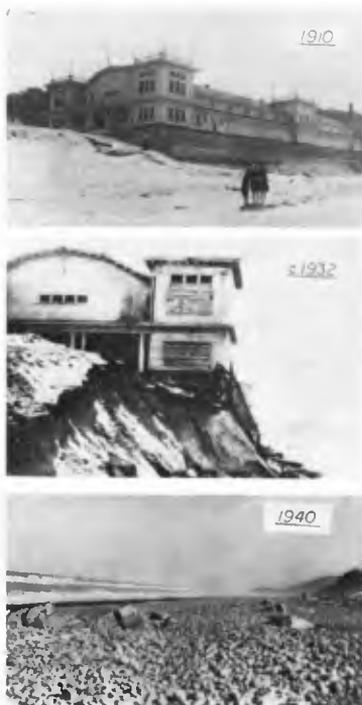
**Figure 3:** Progressive erosion of the natatorium on Bayocean Spit.
