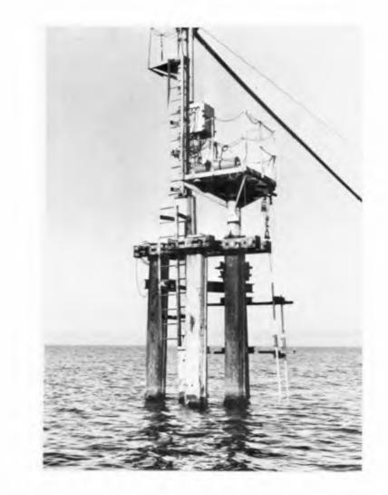
Fig.2. Measuring island with probe installation.
