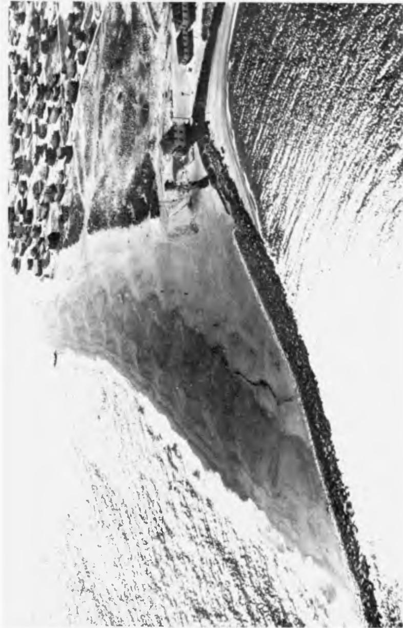
Fig. 3 South jetty of the Merrimack River inlet, Massachusetts, on 16 October 1969. Note the large accumulation and outbuilding of sand behind the Jetty, which was restored in the summer and fall of 1968. View looks south. This is further evidence for local reversal in drift direction on the downdrift side of the inlet. Compare with Figures 1 and 2.
