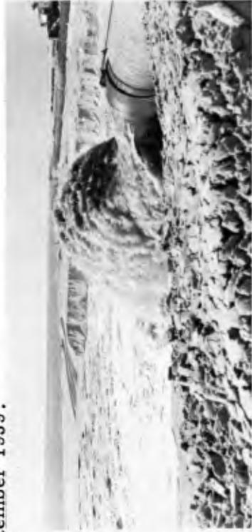
Fig. 15. Discharge from dredge pipeline onto feeder beach.
