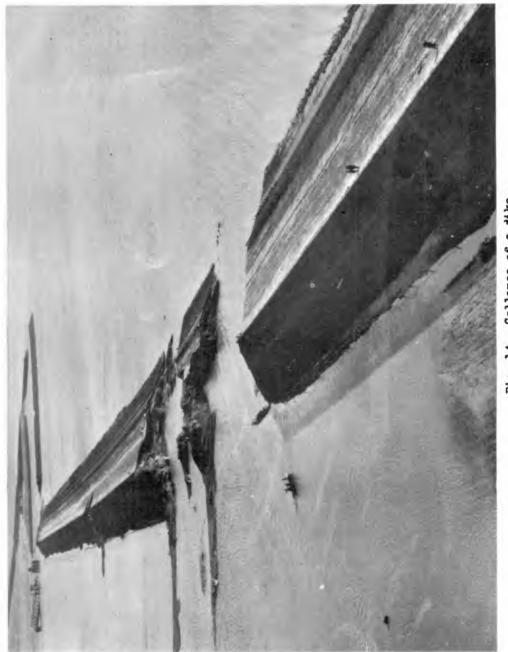
Fig. 14. Collapse of a dike.
