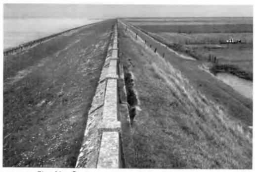
Fig. 12. The first stage of the attack. The fissure on the crest is caused by the strong pressure difference in the ground water.
