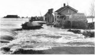
Fig. 18. The tidal currents destroyed the roads in the polders in a short time.
