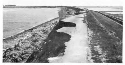
Fig. 11. A damaged dike. The sea is on the right and the land was to the left. Damage occurred at the inner side.
