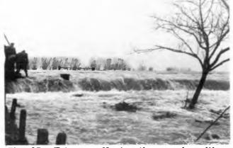
Fig. 17. Water overflowing the secondary dikes.
