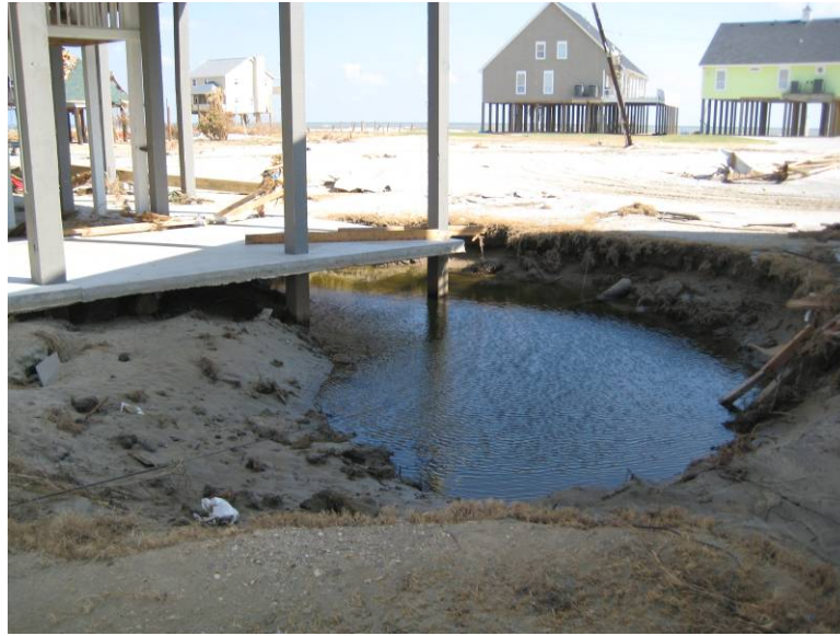
Figure 19 Local scour at the corner of the ground slab
