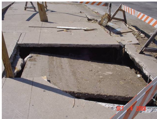
Figure 13 Settlement of slabs behind the seawall caused by piping failures
