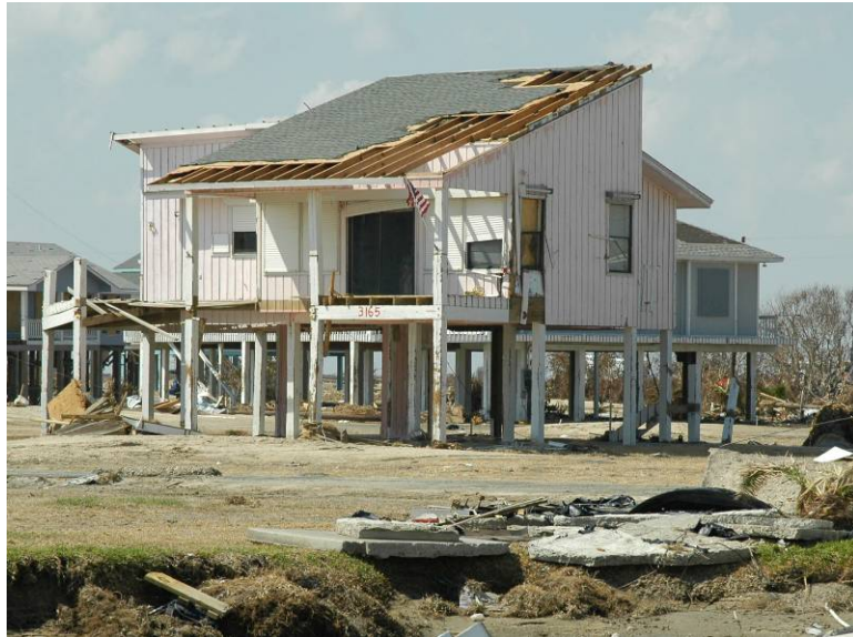
Figure 15 Partial failure of roof deck due to wind uplift
