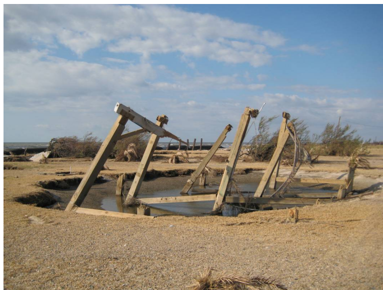
Figure 18 Localized scour engulfing the full footprint of the short pile foundation
