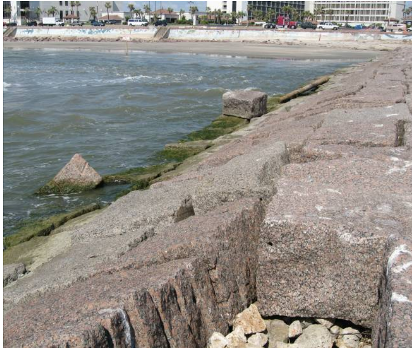
Figure 14 Displaced armor stone at 53rd Street groin
