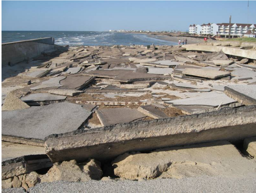
Figure 12 Damage at southwest end of seawall
