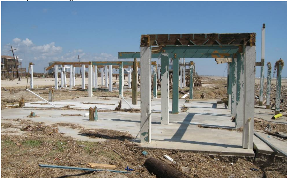
Figure 16 Structural failure due to wave uplift and lateral forcing
