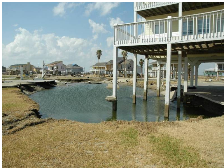
Figure 20 Illustration of growth of scour from slab foundation
