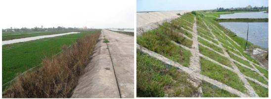
Figure 20. Left: sea dike in Thai Binh with vetiver grass on inner slopes. Right: local grass in concrete frames on Nam Dinh .
